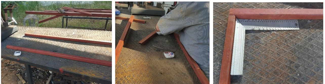
Figure 41 - Marking of Steel Profiles
