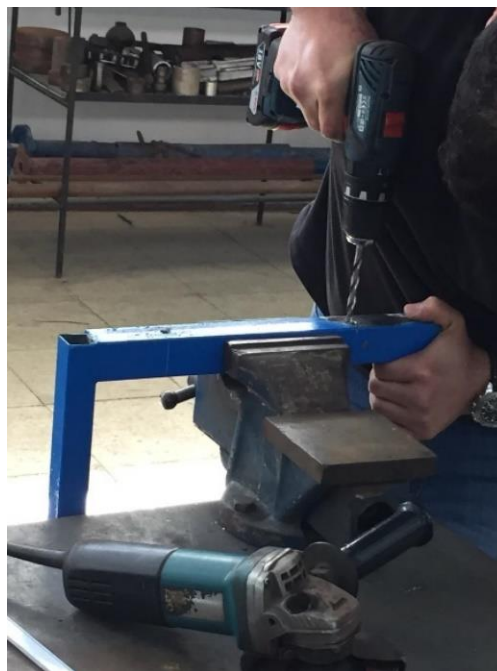
Figure 20: Material removal process of the control system stands using a hand drill.
