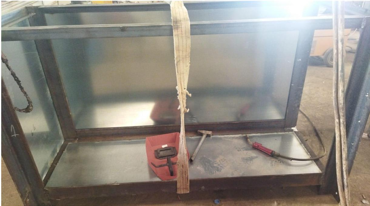
*Figure 42 Welding of galvanised sheets to frame segment*
