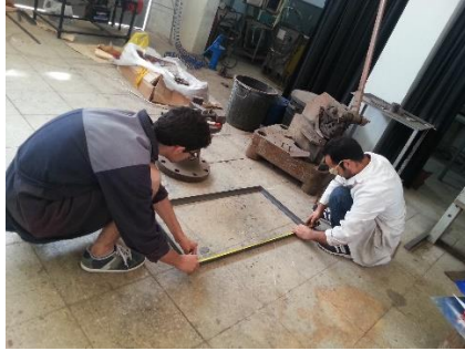
Figure 4.9 Support manufacturing process.
