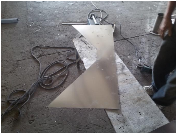
Figure E- 3 Manufacturing air duct wall pt1.
