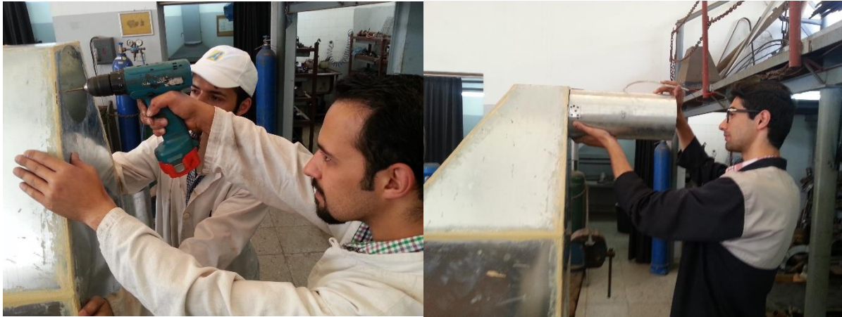
Figure 4.17 Pipe & Air duct assembly.
