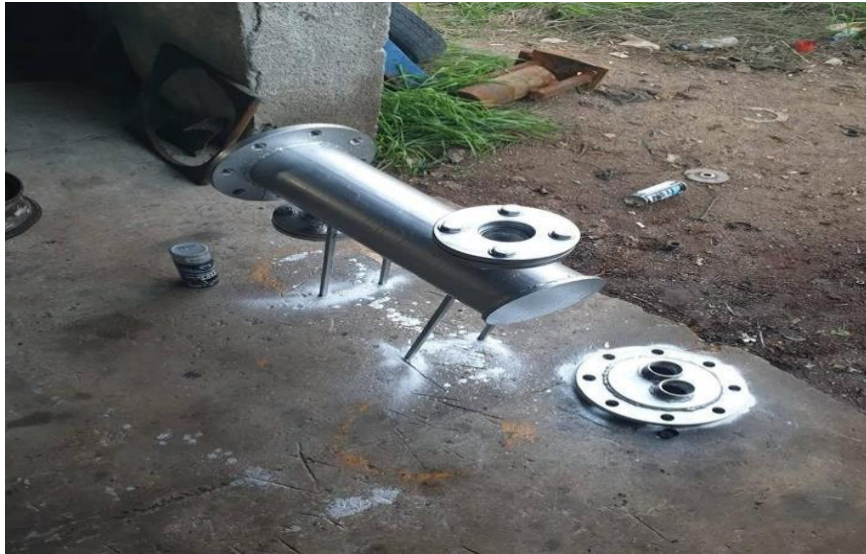
Figure 17 Painting of the shell and tube heat exchanger
