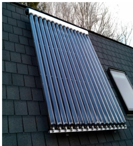
Figure 7. Evacuated Tube Collector [11].
