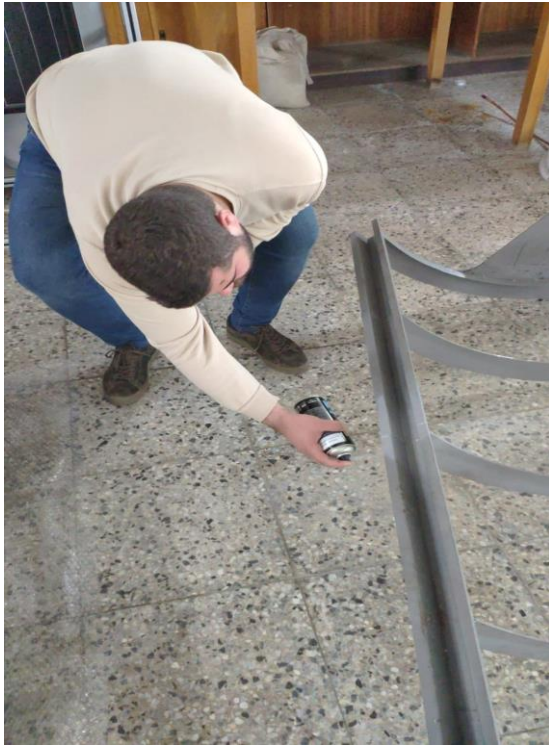
Figure 17. Painting with anti-rust paint
